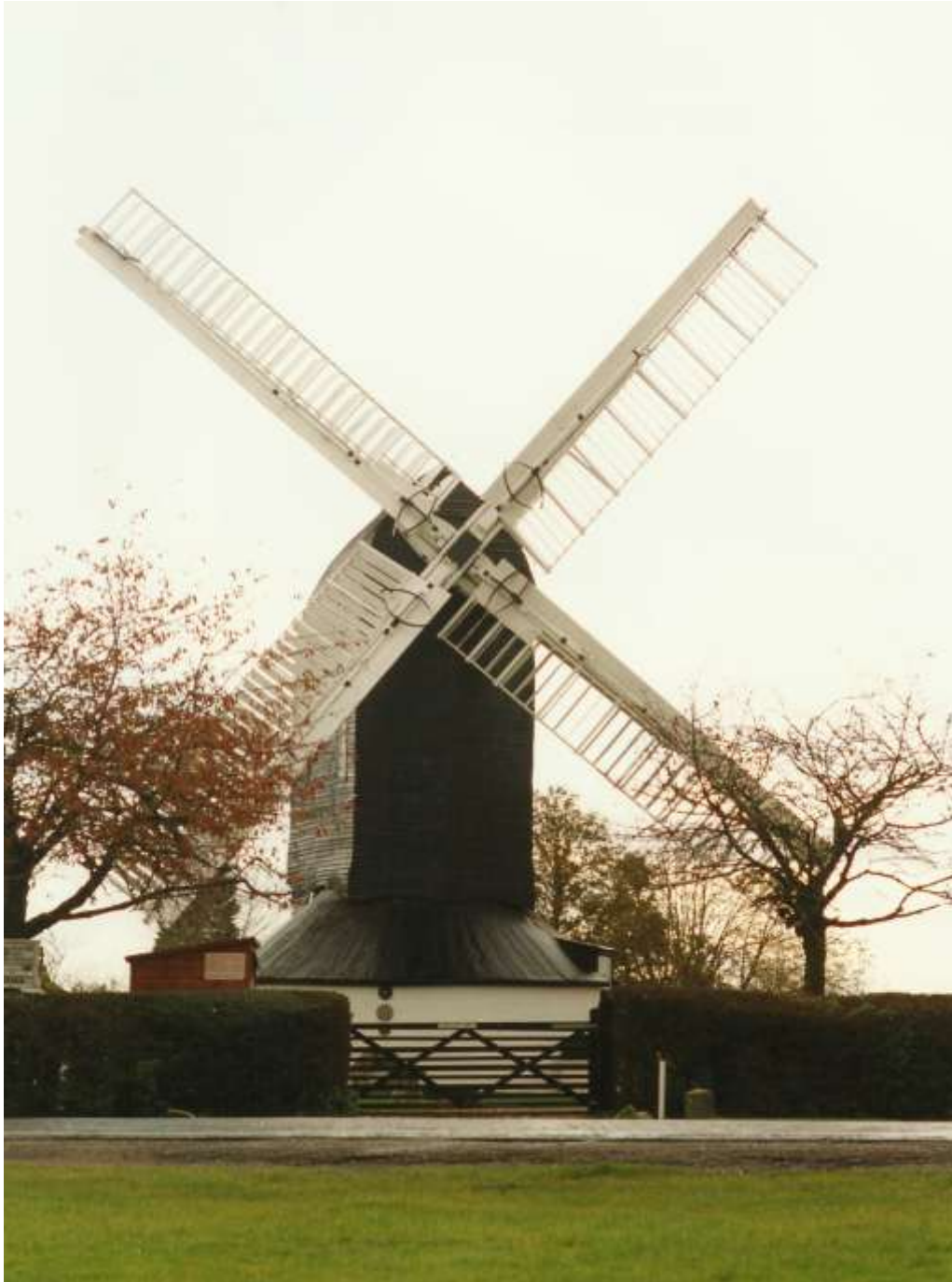
Outwood post mill.
