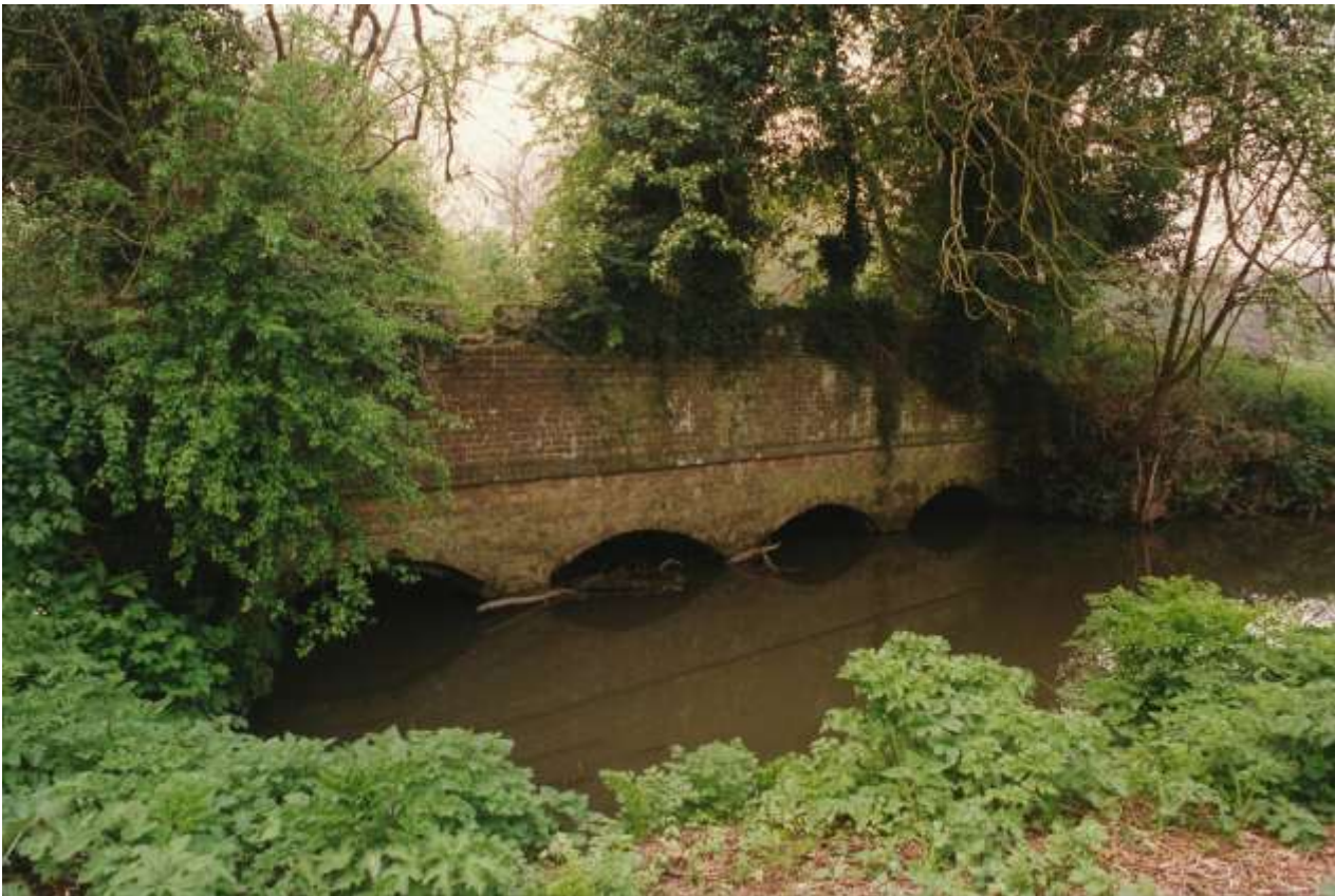
Gosden Common aqueduct carrying the Wey and Arun Canal over the Bramley Brook.
