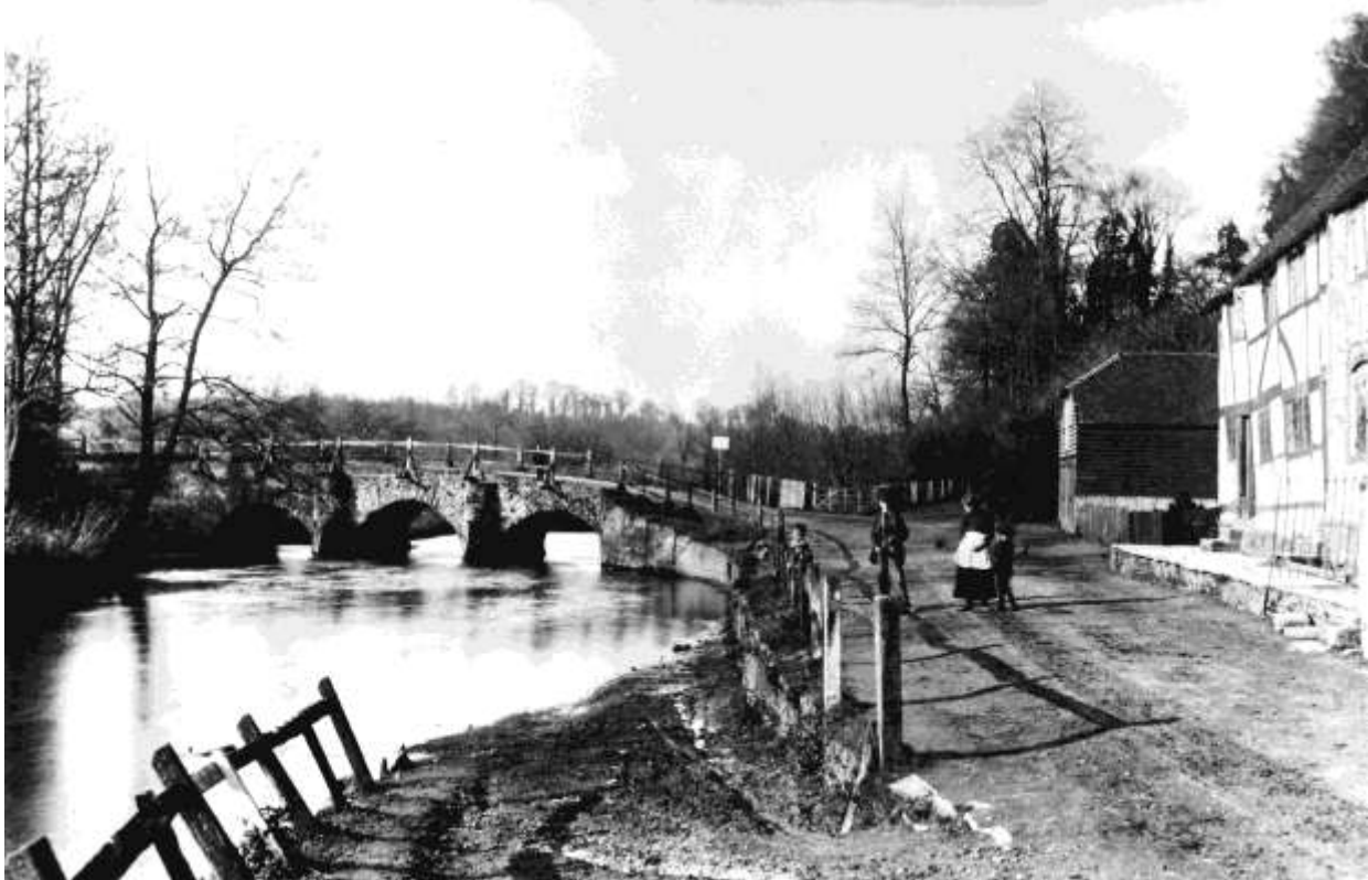
Eashing south bridge, over the millstream, one of a series of medieval bridges on the River Wey, c.1900. Museum of Farnham, John Henry Knight Collection.
